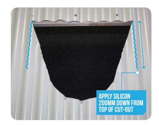
Apply silicon to roof sheeting below flashing.
