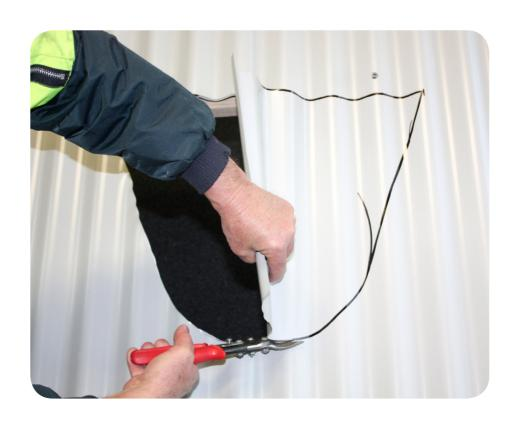
Weather the front of the cut out using pliers to bend the sheet upwards.
